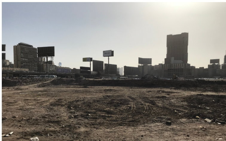
Fig. 2: Maspero triangle after demolition.
